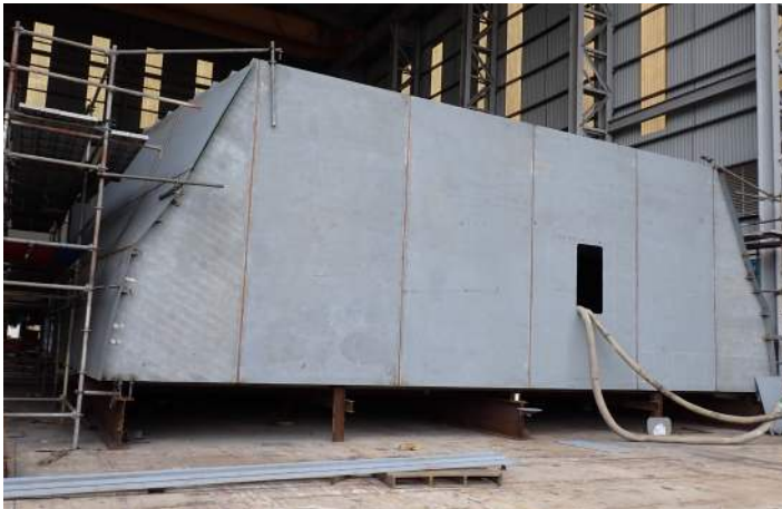
PASSENGER VESSEL | UNIT 7
