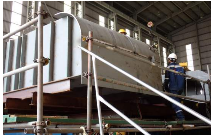
PASSENGER VESSEL | UNIT 7
